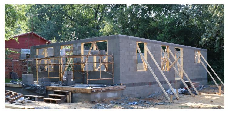
When the emissions were "fed" into the new, lower carbon concrete mix, the result was concrete blocks containing substantially less embodied carbon. The CO2 will remain trapped in that concrete for millennia.
