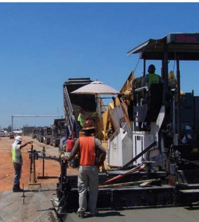
both local and regional concrete industry representatives actively investigated opportunities to utilize Roller Compacted Concrete (RCC) as the pavement of choice at the facility. RCC is a cost competitive, long-term paving option which takes its name from the construction method used to build it. RCC is typically placed with high density paving equipment and compacted with vibratory rollers. Paving widths of 30 feet wide at a ten inch depth are possible in a single pass.
