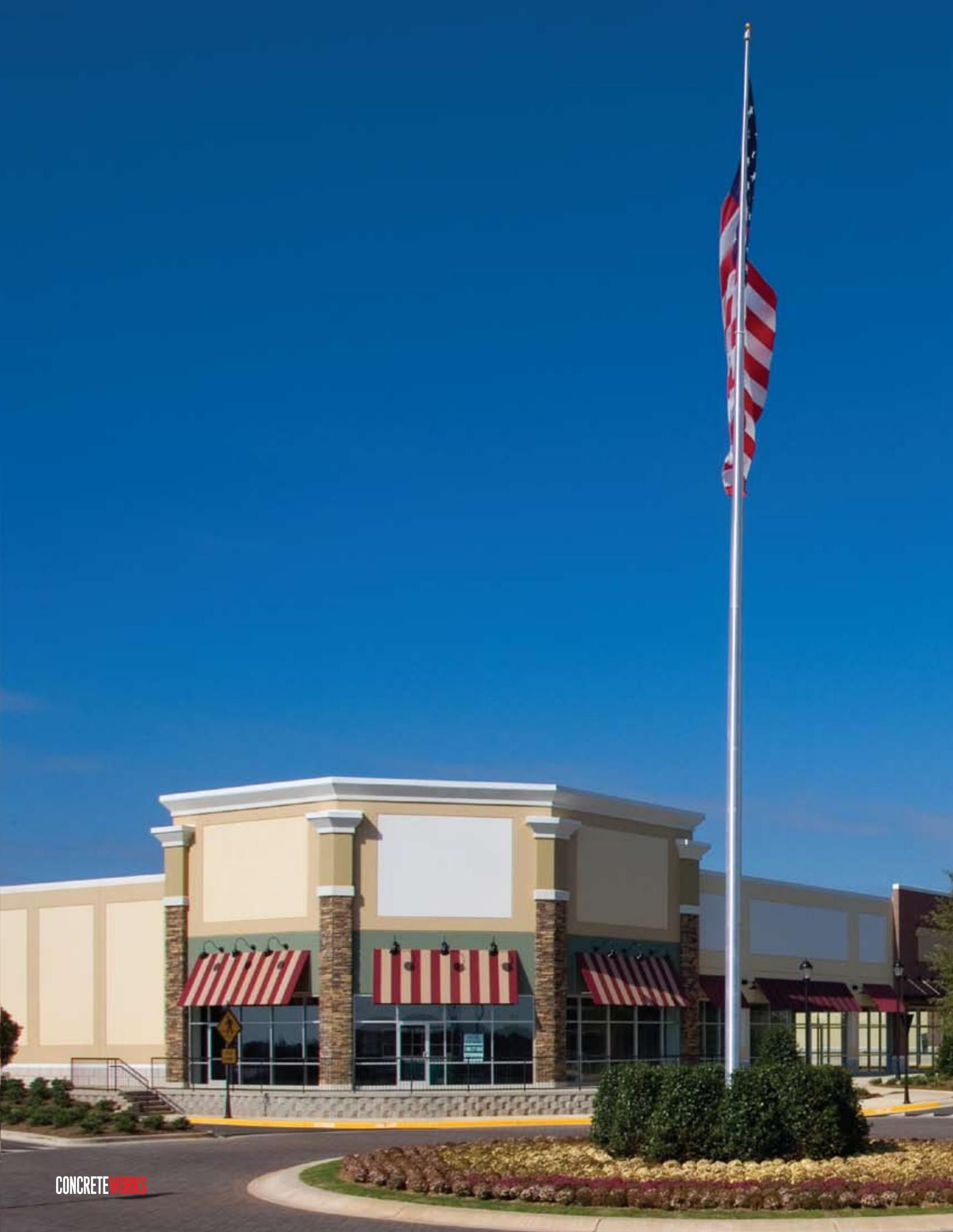
The panels were set to keep architectural features from conventional construction into tilt-up. The complexity of the panels set new standards in the tilt-up construction industry.
